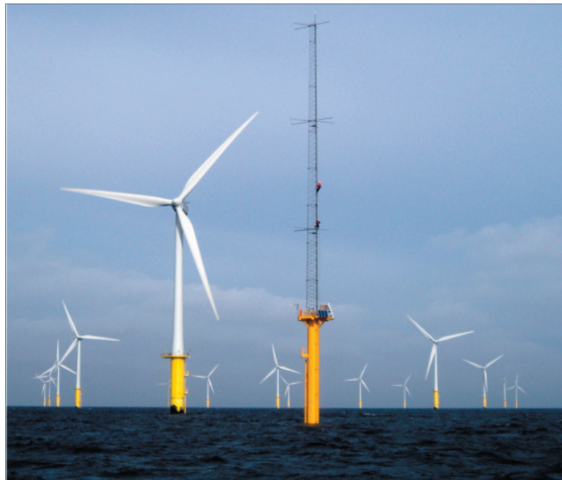
A Campbell Scientific datalogging system monitors this offshore wind farm located between Rhyl and Prestatyn in North Wales at about 7 to 8 km out to sea (photo courtesy RADTech Ltd. UK).
