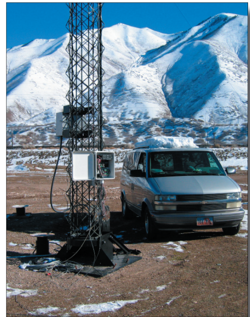
This wind assessment site uses a Campbell Scientific data acquisition system to collect data from an IsoTruss tower and sensors.
